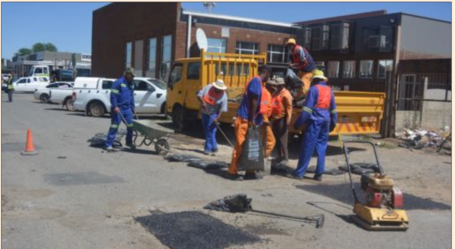
Pothole patching in Delareyville in Tswaing Local Municipality, Ngaka Modiri Molema District as part of Setsokotsane 10 x 10 campaign.
